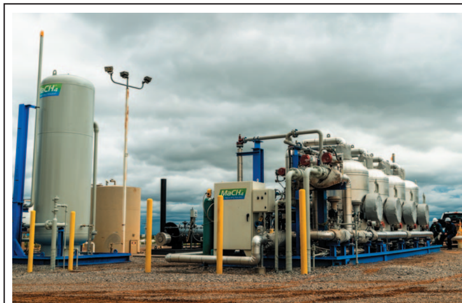
Coldstream Energy's MaCH4 fuel-gas treatment system removes natural gas liquids from the fuel stream, allowing operators to retain and sell NGLs that otherwise would be burned as fuel. The company says the technology reduces emissions, improves engine reliability and can generate substantial additional revenue.
